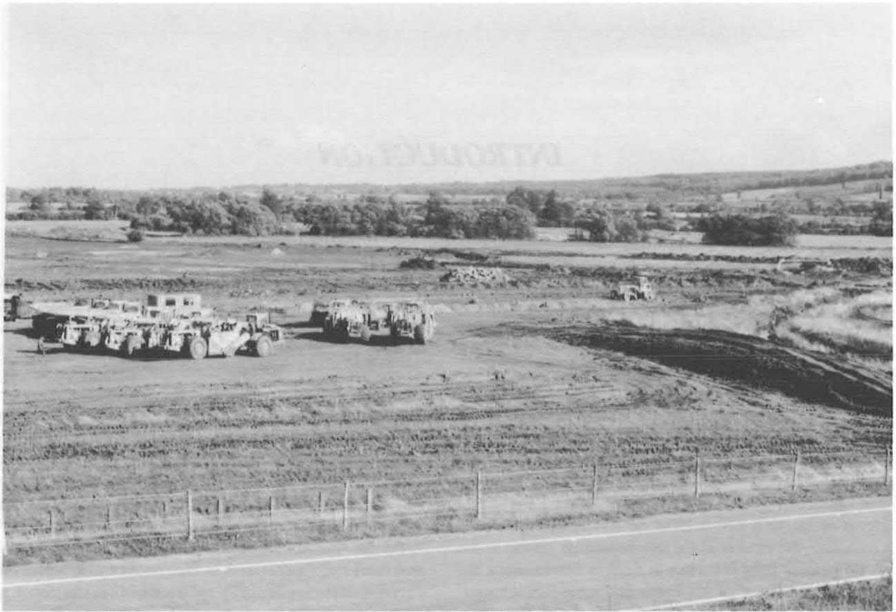
Plate 1: Construction of Caldecotte Lake, 1981 (MKAU).
